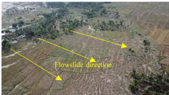
(b) Many significant cracks appeared in downslope area of the flowslide
